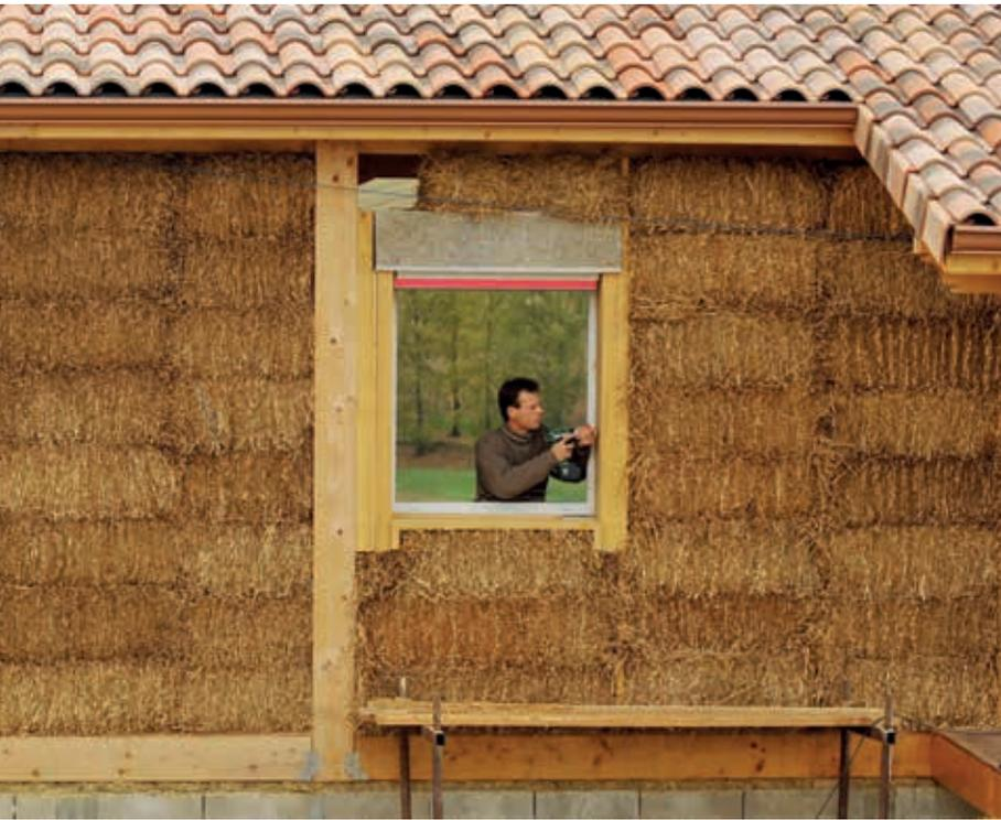
**E** Compressed hay used in construction can bear heavy loads, provides great isolation and resistance against earthquakes and fire.
